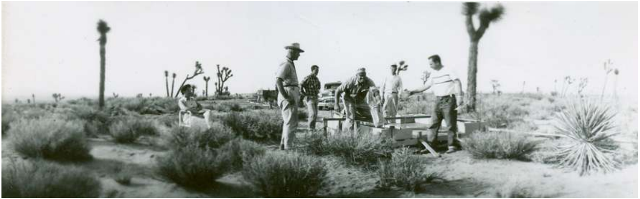
Generator and tool room foundation start.
