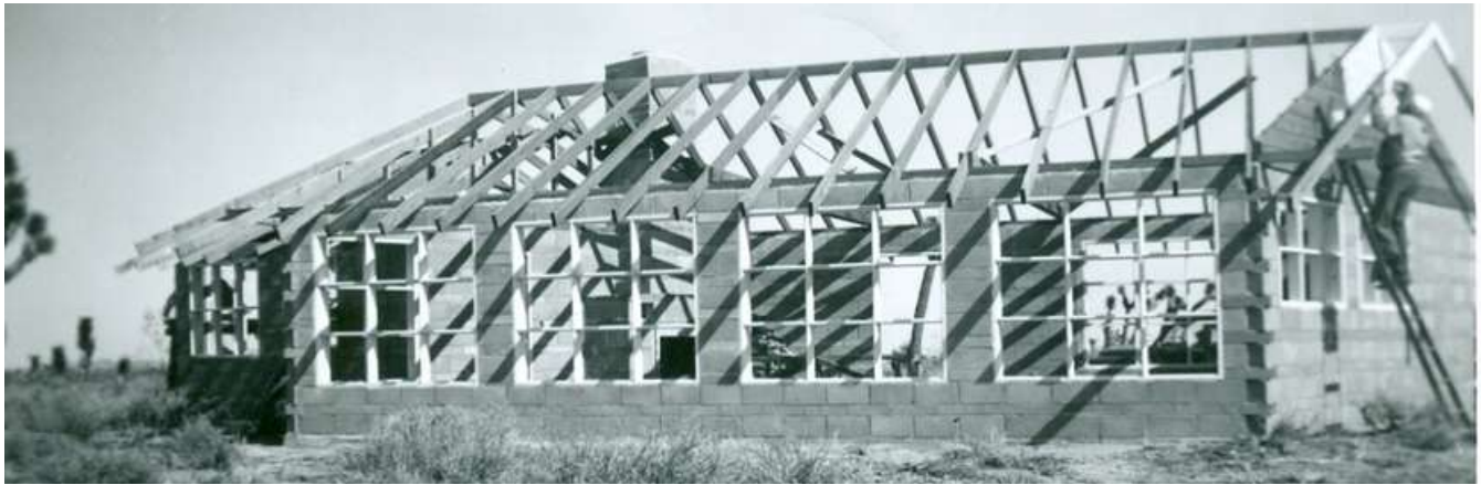
West side of our Desert House under construction fall 1950.
