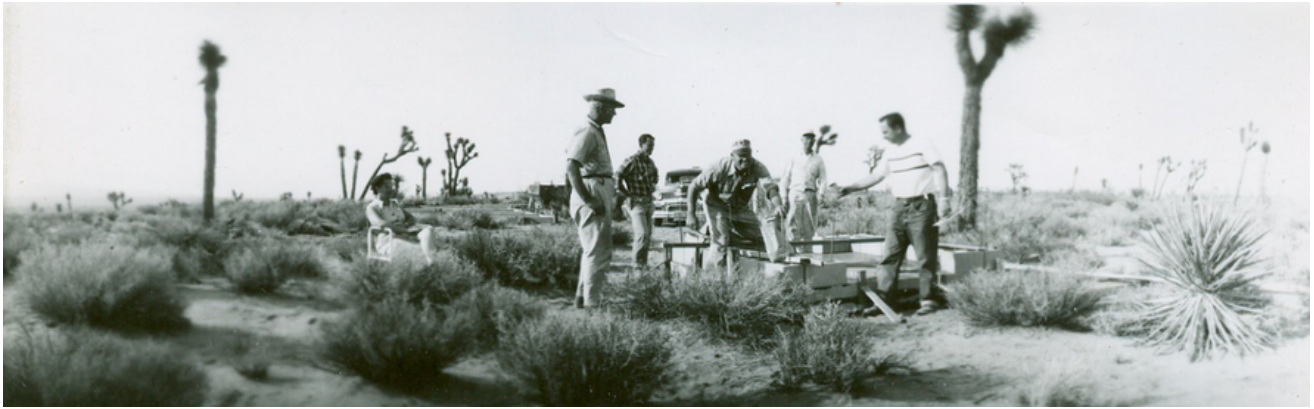
Generator and tool room foundation start.
